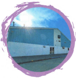
Heating & Air Upgrades Petersburg Community Foundation
